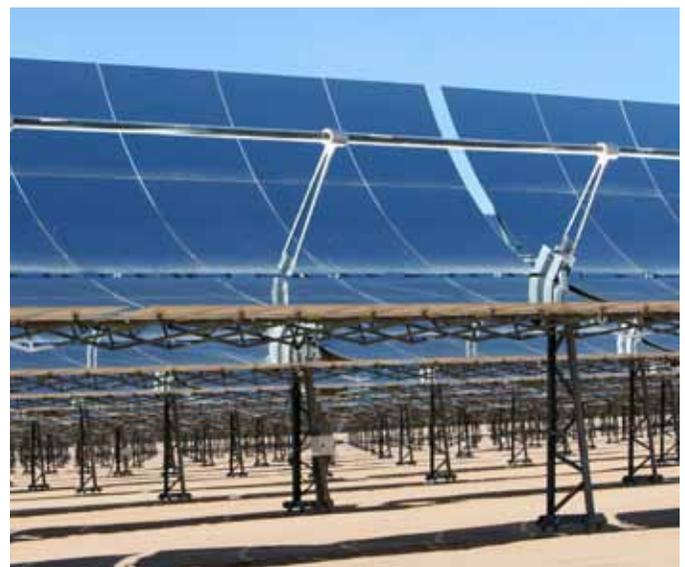
Illustration 3. Parabolic trough solar concentrators
